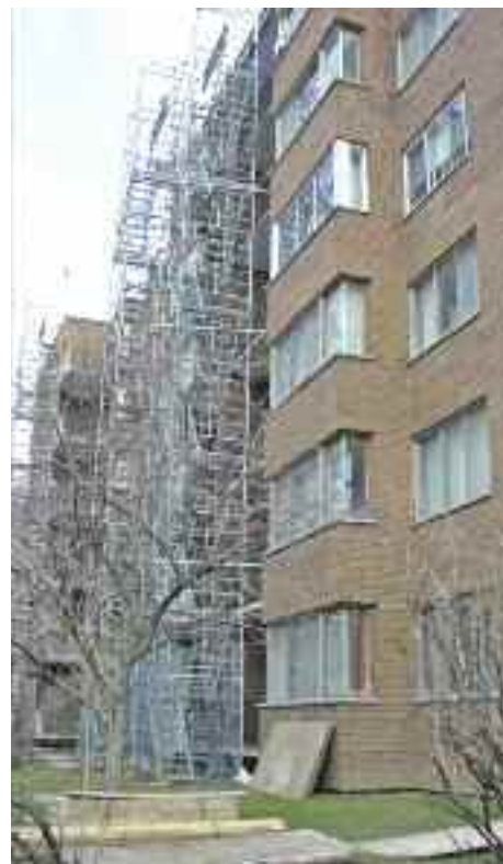
Replacing balconies at 400 Lansdowne.
