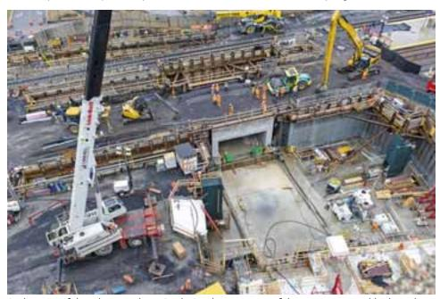
At the time of this photograph on April 20, a large section of the concrete tunnel had just been pulled into place. The Glen hospital is to the south, at the top of the picture. Photo: RALPH THOMPSON.
