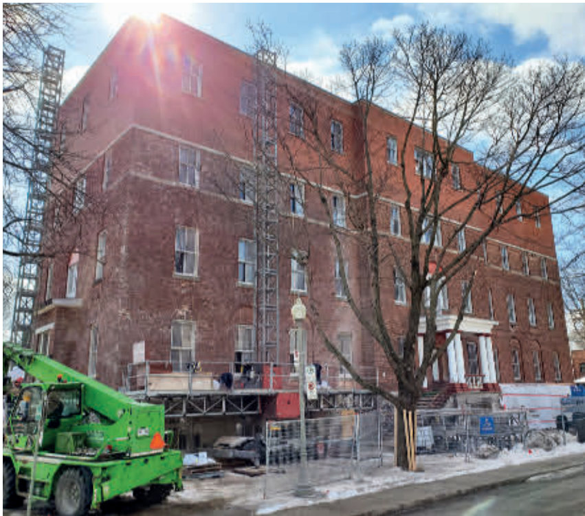
Workers were busy re-pointing the brickwork at 500 Claremont March 16, using scaffolding that is new since our January visit (see January 18, p. 7). The building is to be rental apartments when finished.
