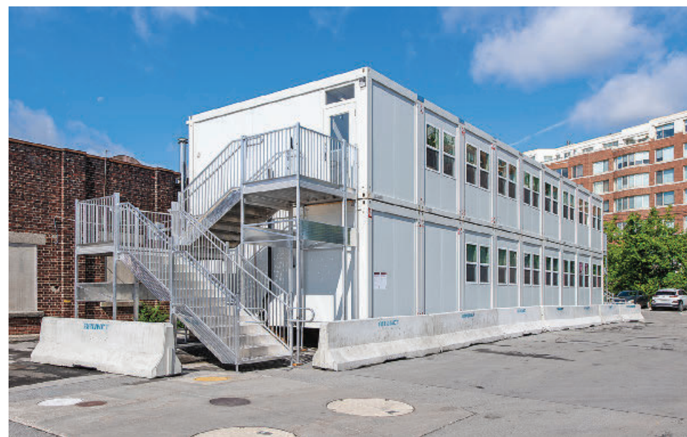
Temporary cabins have been set up to accommodate workers during the renovations.
