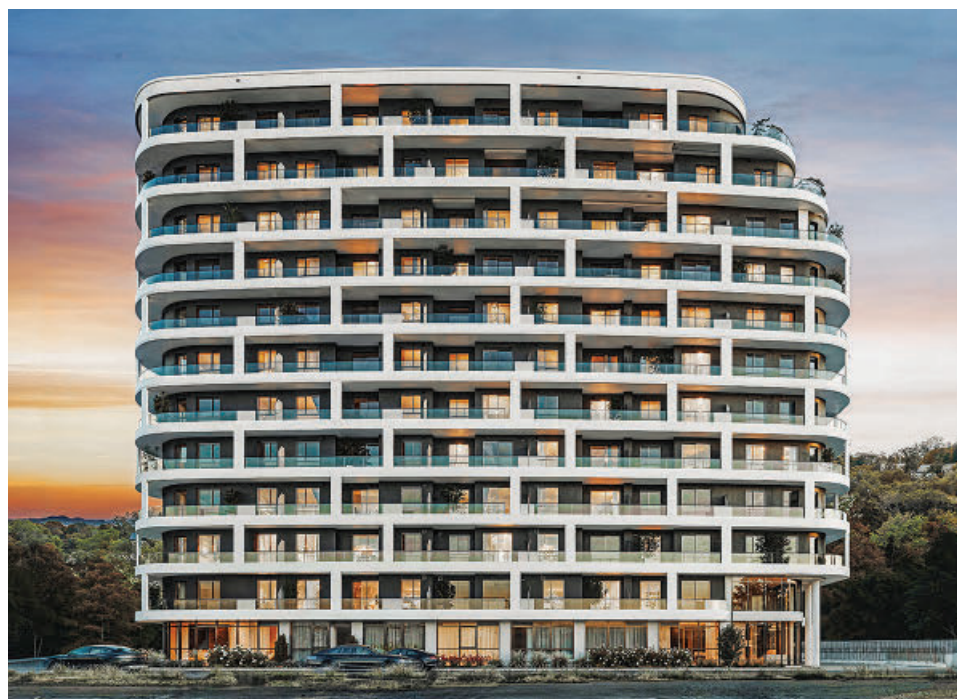
The planned apartment building Le Loyal is under construction at 4845 Côte St. Luc Rd. It is outside of Westmount, to the northwest of the city.
