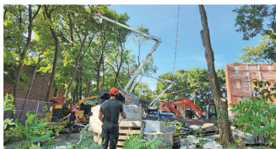
Two tree crews at work simultaneously at 500 Claremont on September 6.
