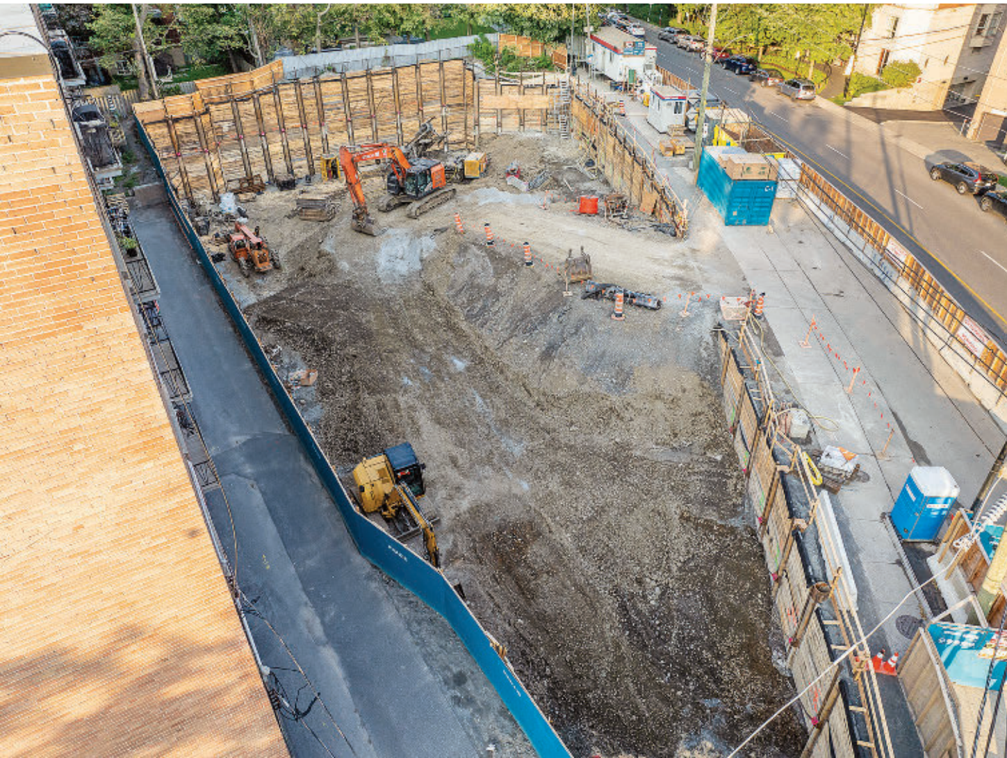
A view of Le Loyal's worksite, as seen September 11.
