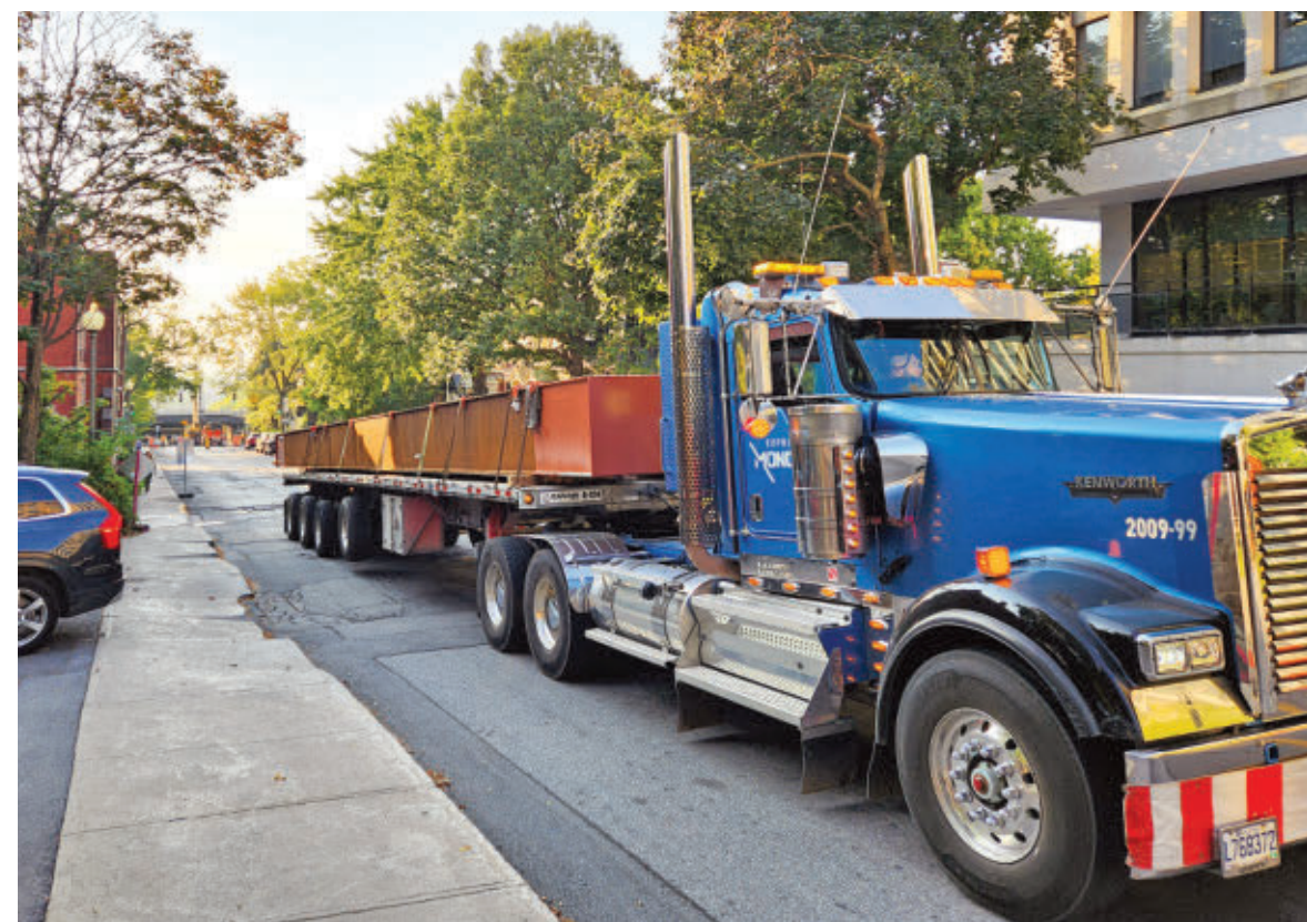
Left, protective beams being backed down Greene from Dorchester the morning of September 13. The car at left was unceremoniously and rapidly hustled by a flagman onto the private parking pad on the east side of the street. Right, the crane waiting for its payload. As previously reported (see October 17, 2023, p. 1), the idea is to protect the CP rail bridge over Greene from truck strikes, of which the Independent has chronicled at least 18 of the roughly 30 since November 2020.
