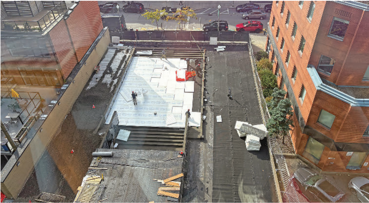
Looking down at the laying of the exterior plaza membrane over the Greene entrance to Westmount Square. As seen on November 4.
