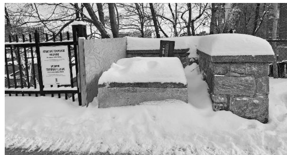
The steps from Stanton St. up to Thornhill Ave. have been closed for months, as seen February 7 from the top.
