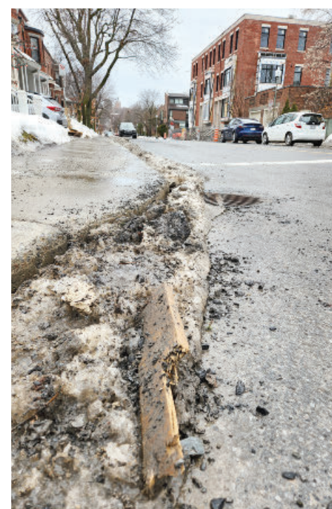
On March 3, there was still some lumber debris in the area.
