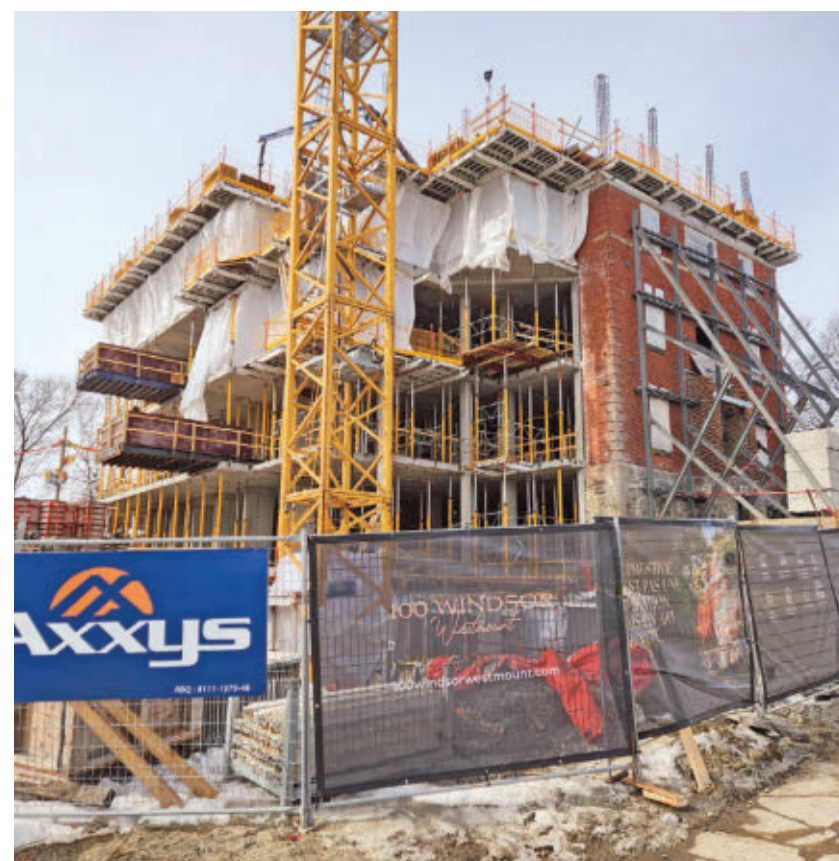
The 500 Claremont apartment development/conversion was a bustling and bristling worksite March 13.
