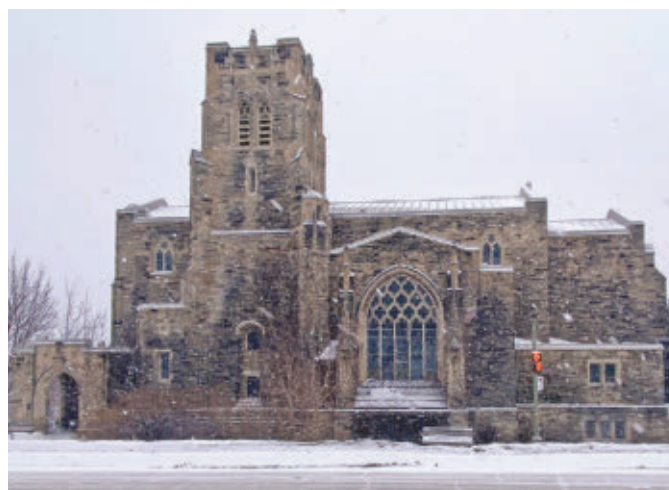
The former Mountainside United Church is on The Boulevard between Roslyn and Lansdowne avenues. Photo taken on February 27.
