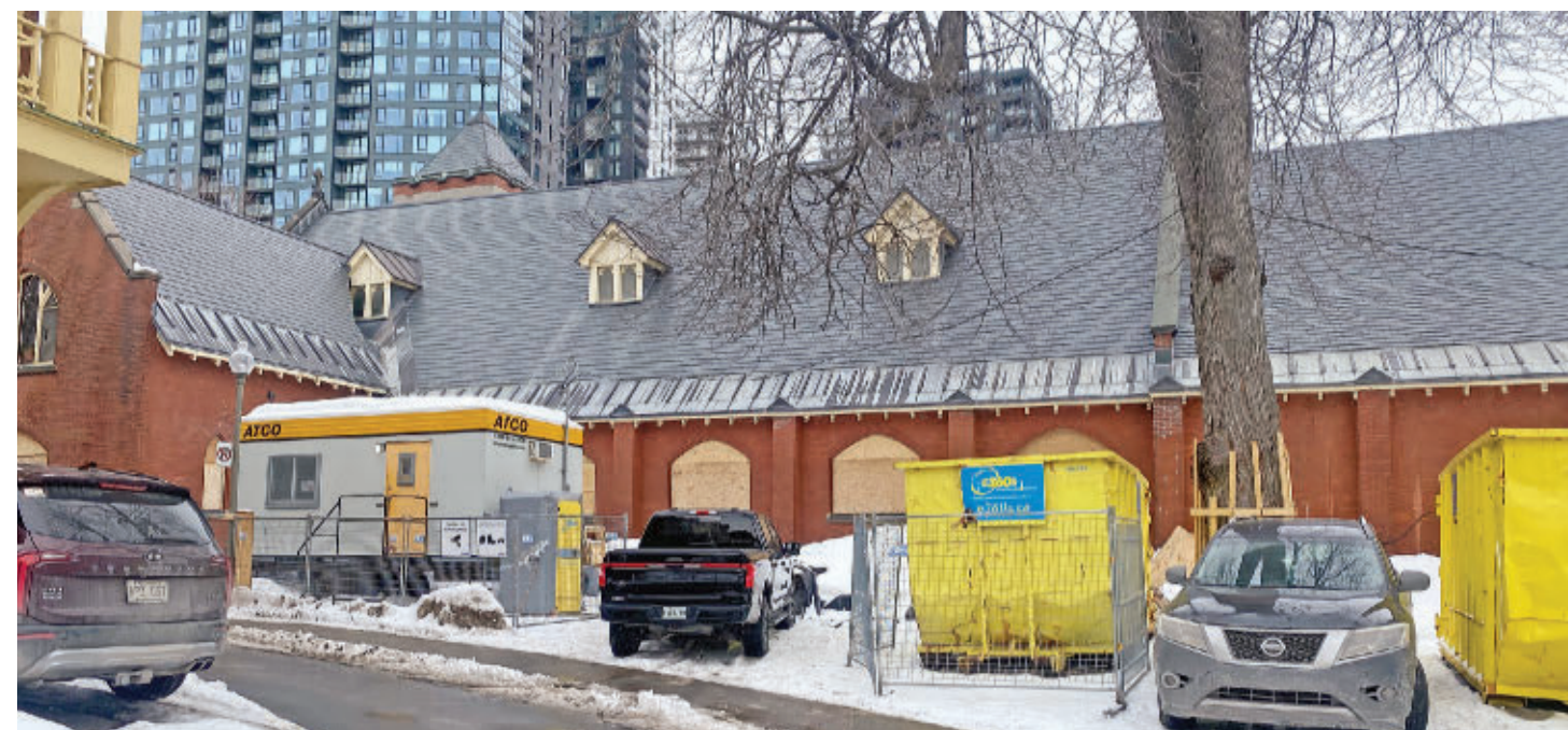
The west side of the former St. Stephen's Church, as photographed looking east from Weredale Park road on March 4.
