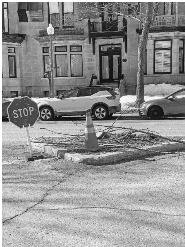
The temporary stop sign at Wood and de Casson on March 19.
