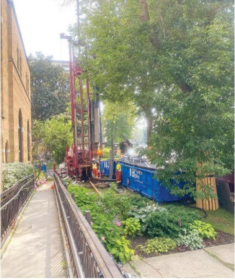
Drilling the first well for Temple's geothermal climate control system on July 14.
