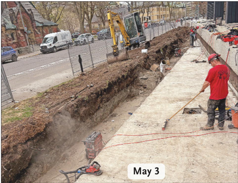
The sprinkler system was ripped out at de Maisonneuve and Greene Ave. to replace the water membrane. As seen on May 3.
