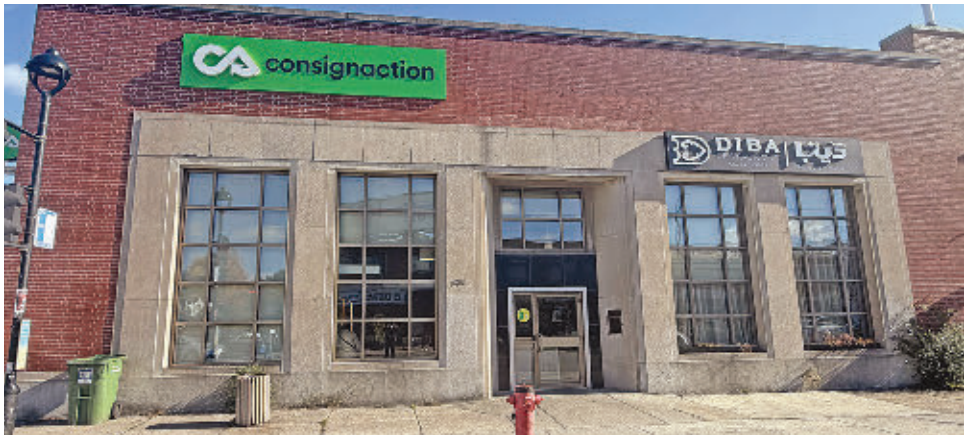
Consignaction at 6510 Somerled Ave. near Cavendish.
