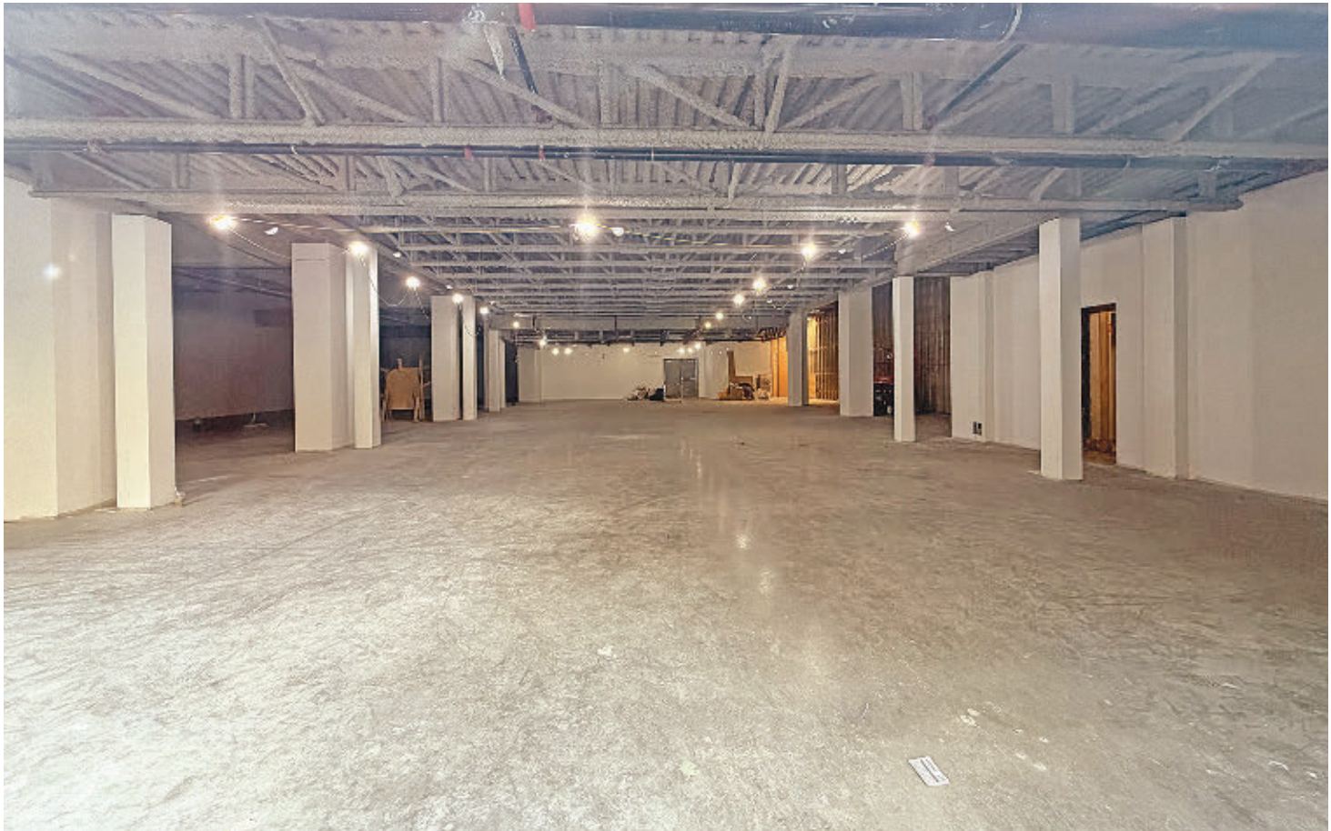
5024-38 Sherbrooke is one lot of three buildings owned by 2964 0968 Quebec Inc. Looking through a window into the worksite indicated that the ceiling is completed as well as the flooring, as seen October 6.
