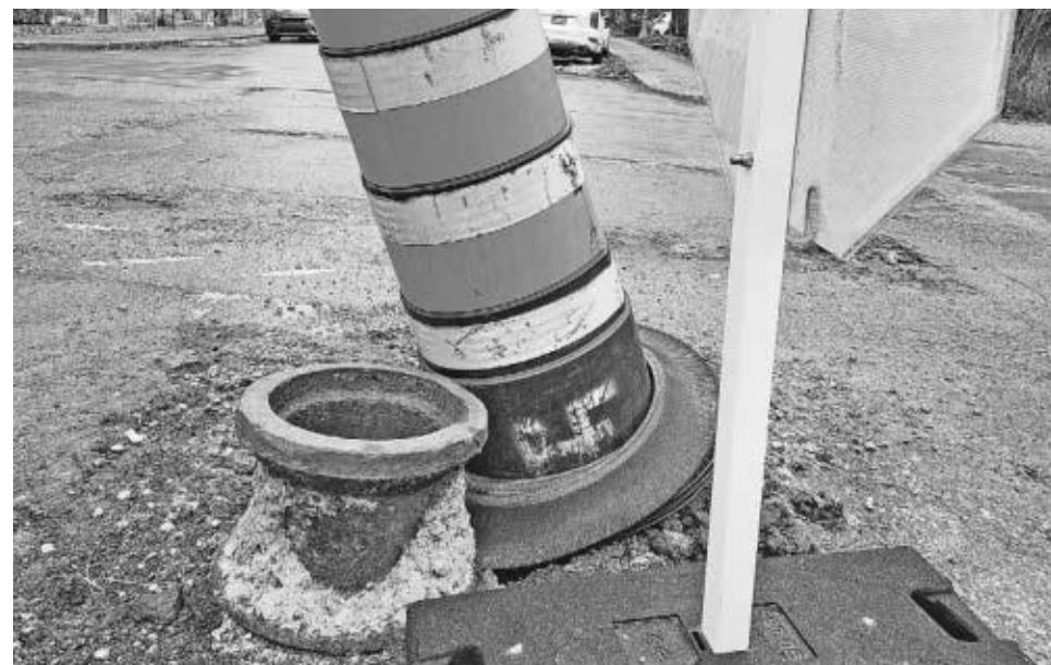
As seen at Prince Albert Ave. and de Maisonneuve March 31. This metal joint of some kind was there for many days, but had been removed by April 20, although an orange cone was still in place.
