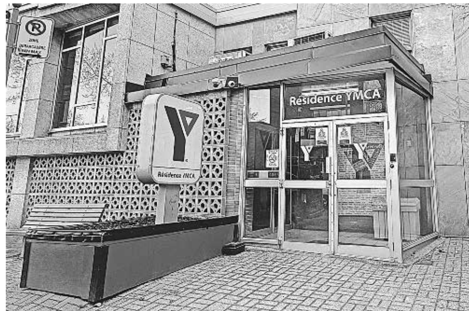
The YMCA residence is located at 4039 Tupper St., as seen April 9.
