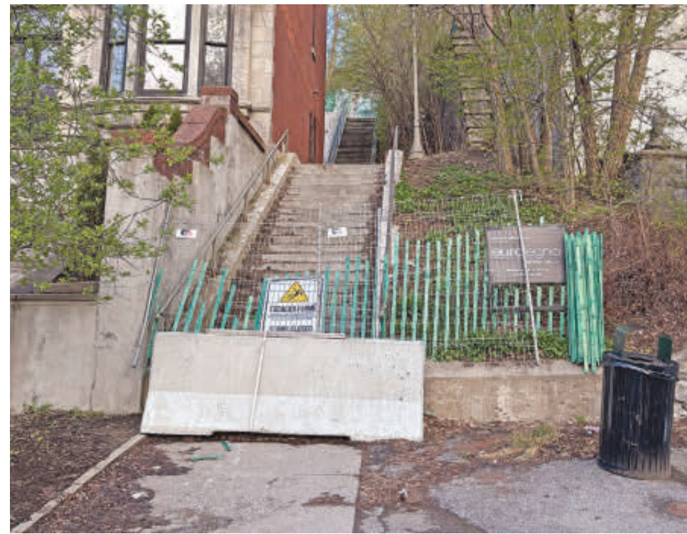
The staircase connecting Holton Ave. to Mount Pleasant Ave. on May 7.
