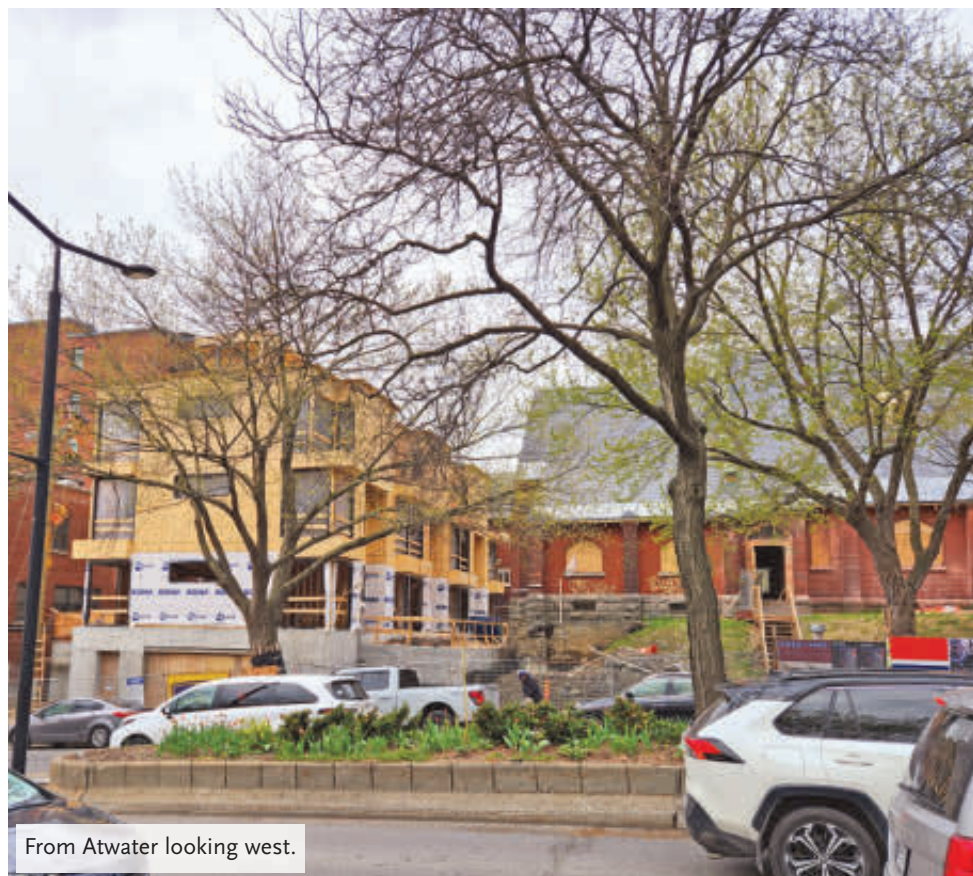
From Weredale Park road looking southeast.
