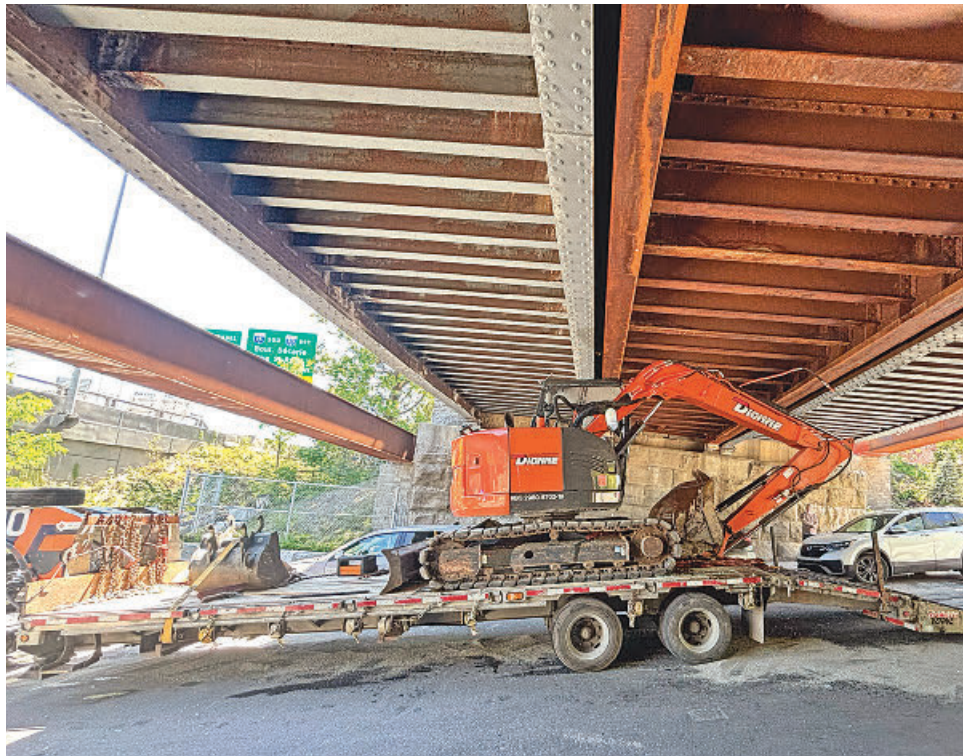
According to the Independent's unscientific records, the rail bridge over Greene Ave. below Dorchester is more often hit from the St. Antoine/northbound side, as it was on June 1 and 5 (not pictured). This southbound digger was caught by some combination of the protective I-beam and the bridge itself on June 3.
