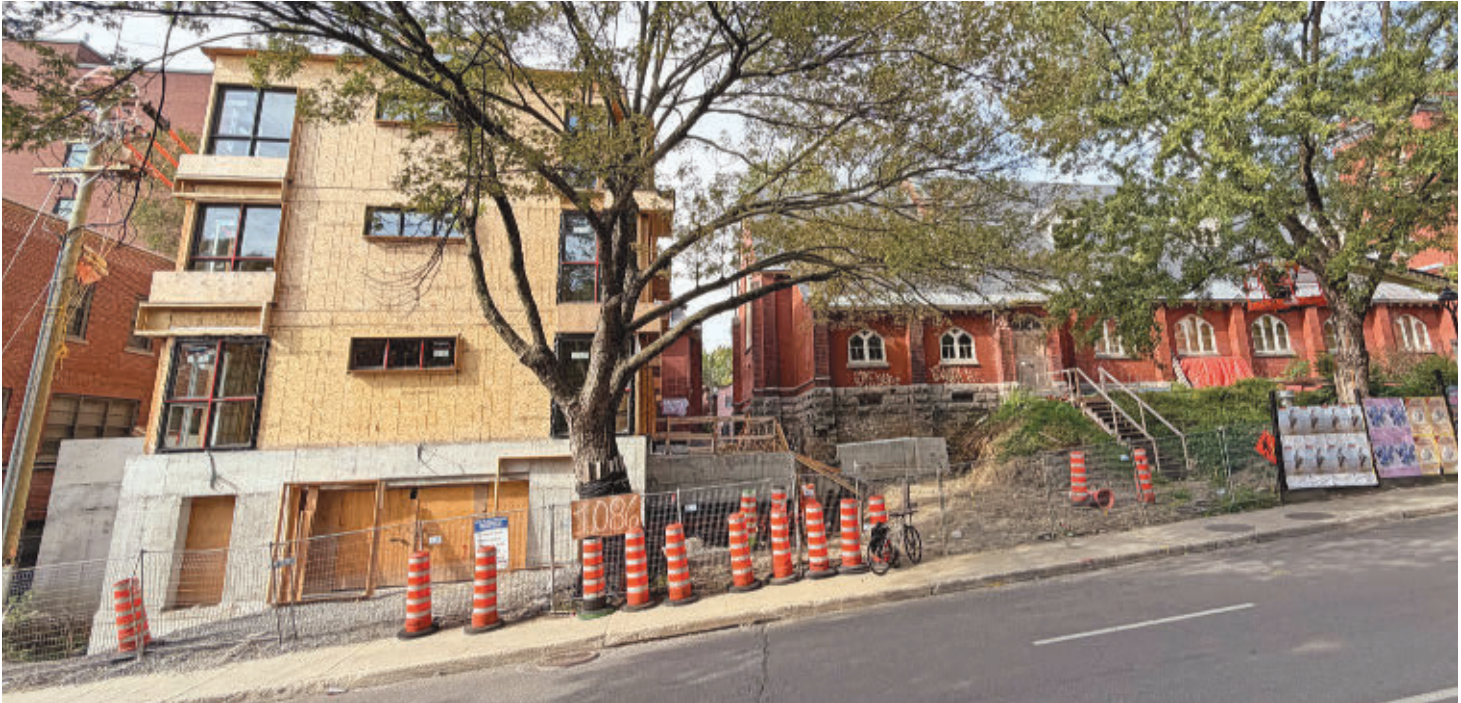
This view from Atwater Ave. looking west shows the former St. Stephen’s church, right, and new a low-rise building, left, still under construction. The newly constructed four-storey building will have nine units and the existing church will have five. Photo taken August 30.
