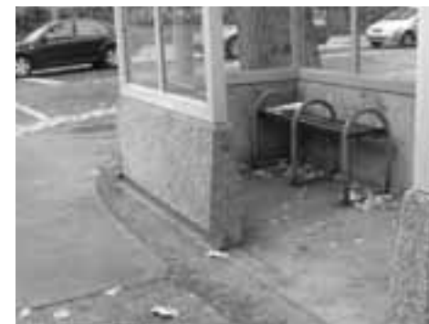
Southwest corner of Wood.
