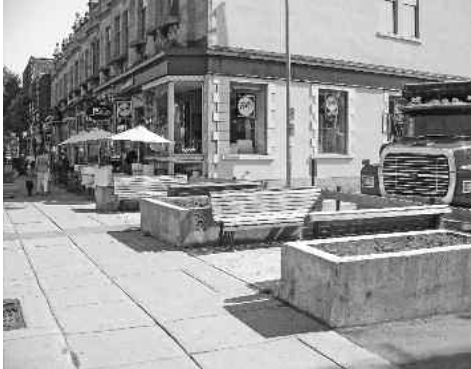
Site of the new Prince Albert square, September 5, before the start of work.
