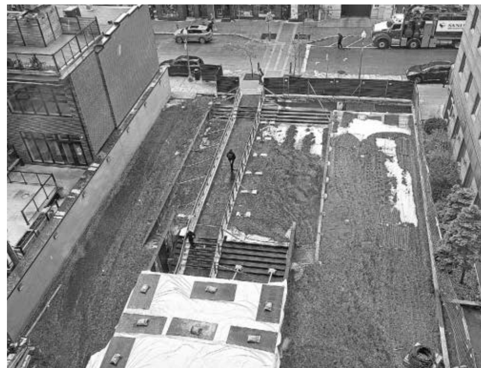
Temporary access to Westmount Square's concourse and its tunnel to Alexis Nihon opened on November 27, 2025, as seen the same day.
